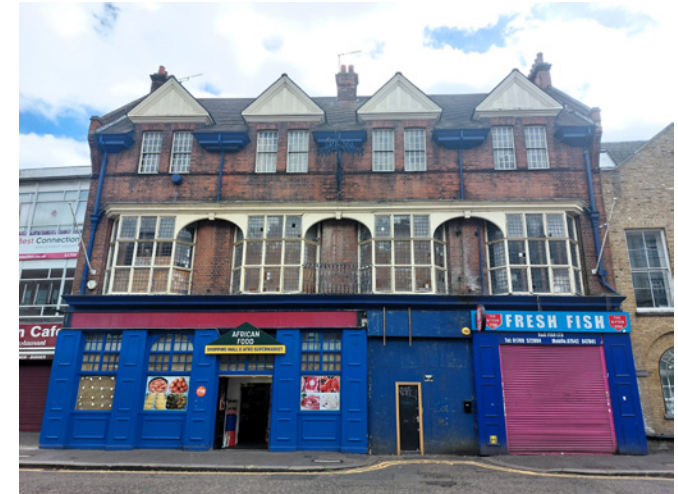
Brickwork and glazing damage to locally-listed White Hart façade on the High Street
